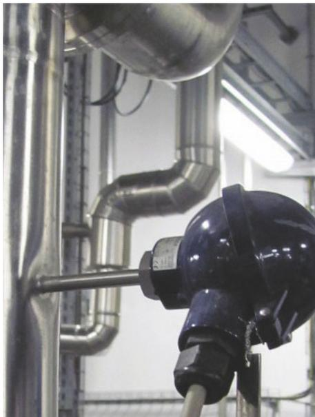
Resistance thermometer for orbital welding
